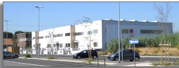
Assemblad – new operative headquarters
